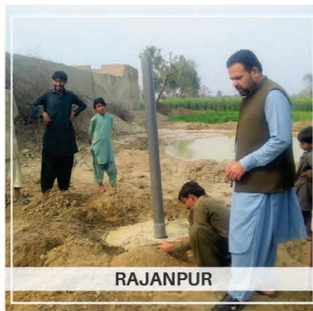
Installation of Deep Well Afridev Hand Pump at Village Allah Buksh
