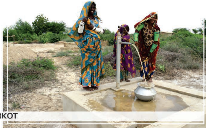
Communities of Village Ayaz Rind are benefiting from the installation of Hand Pump
